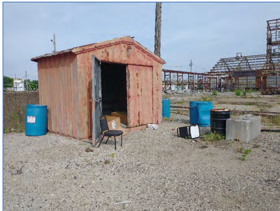
Photo 6: Fire Shed with Foam Drums
