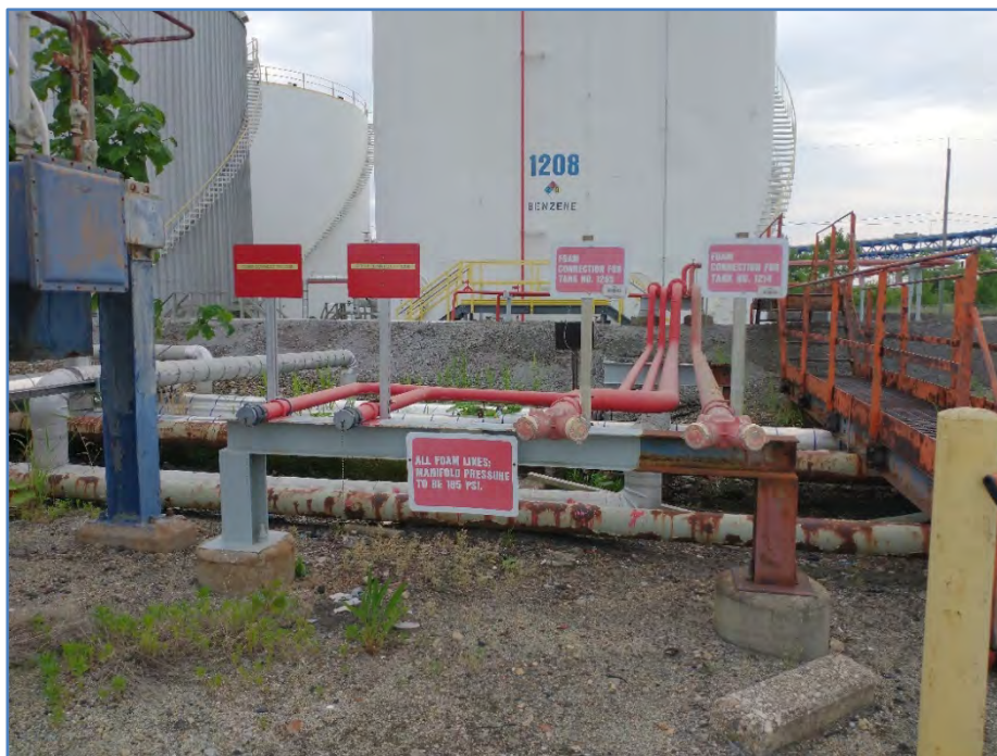
Photo 8: Foam Loading Area-1200 Tanks
